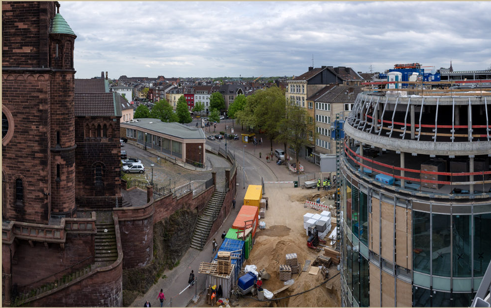
Picture of the week 2015 (21), Baustelle Aquis Plaza, Aachen, Mai 2015
